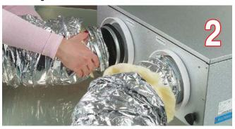
Cover the air handling unit spigots with the inner hoses of the heat-insulated air ducts and fix those with metal clamps (special accessory).
