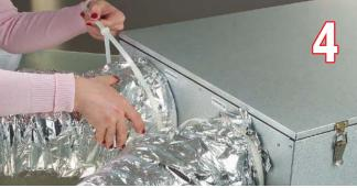
Cover the flanges of **NM Isovent** mounting kit with inner hoses of heat-insulated air ducts by pressing the hoses tightly against the air handling unit casing and fixing those with clamps (included into delivery).
