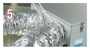
■ Tighten the connection point between the inner hose of the heat-insulated air ducts and the flanges of **NM Isovent** mounting kit with clamps.
