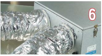
Heat-insulated air ducts have reliable connection to the air handling unit spigots
