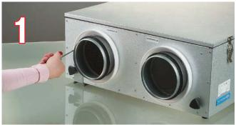
Cover the air handling unit spigots with the flanges from **NM Isovent** mounting kit and fix those with self-drilling screws with hexagon washer head.
