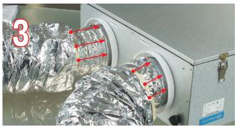
Tuck the inner insulation layer of the air ducts under the flanges of **NM Isovent** mounting kit.
