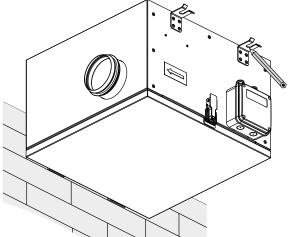
**3.** Fix the fan on the mounting brackets using the appropriate fasteners.
