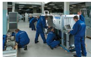
AirVents air handling unit workshop
