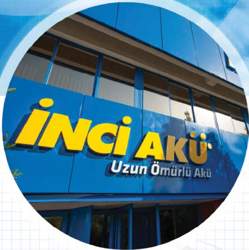
İNCİ AKÜ BATTERY FACTORY Izmir, Turkey
