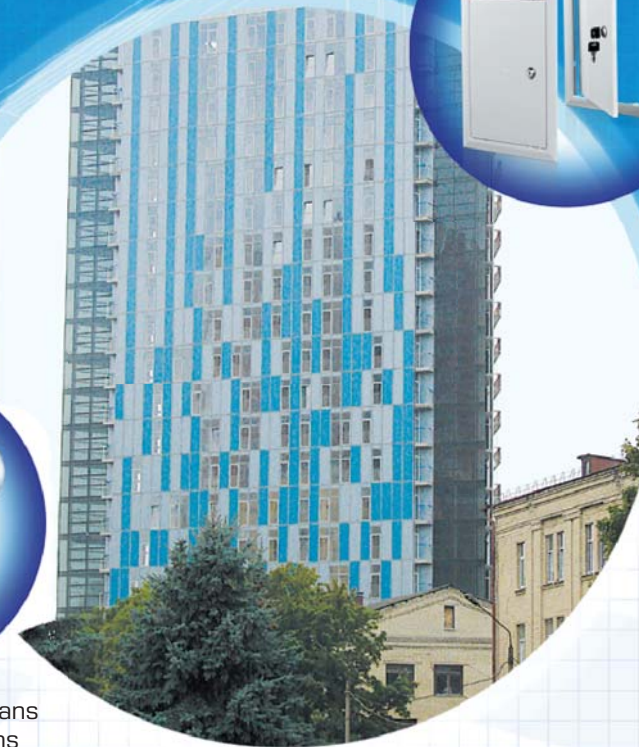
RESIDENTIAL BUILDING 18 a Otakara Yarosha St., Kharkiv
