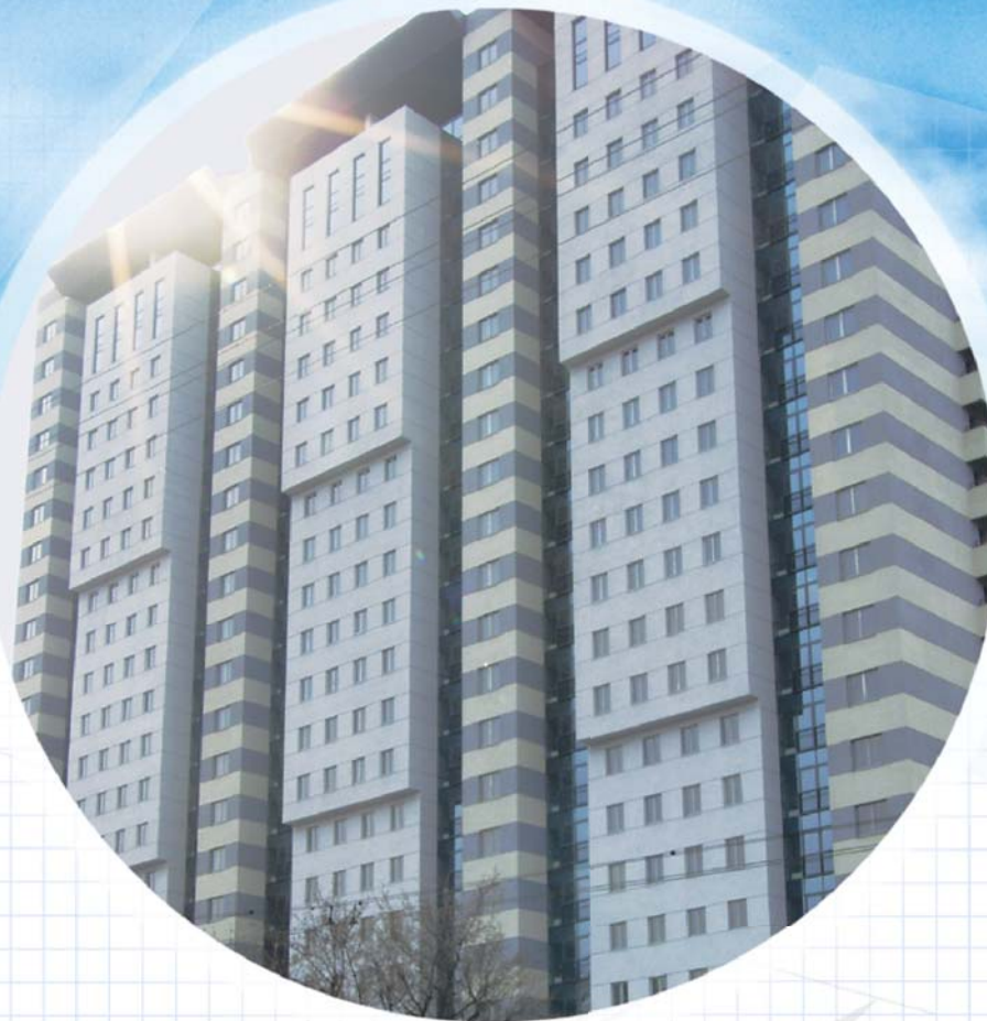
RESIDENTIAL BUILDING 18 a M. Loyana St., Dnipro
