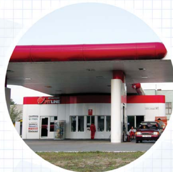
YUKON PETROL STATION
