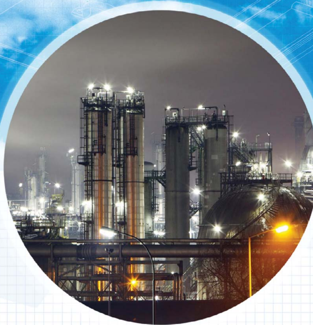
DYO PAINT FACTORY Izmir, Turkey
