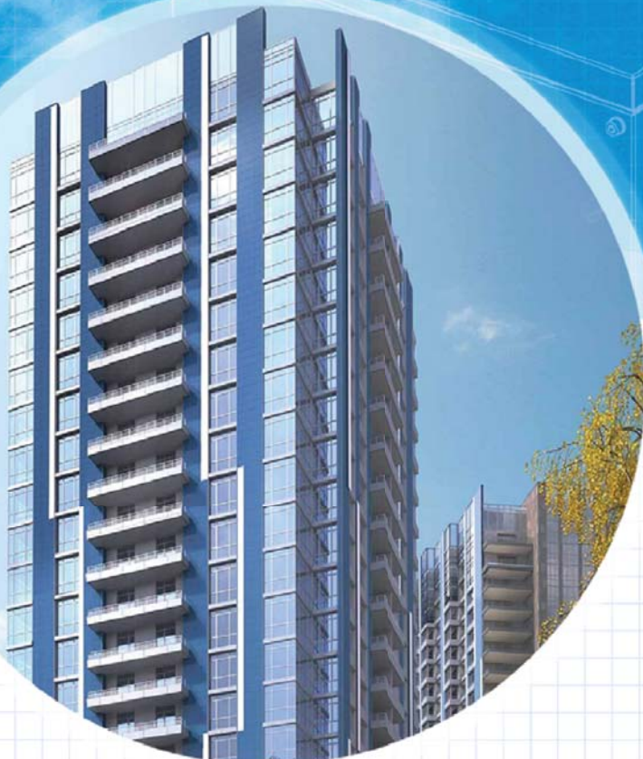
CENTRAL PARK RESIDENTIAL COMPLEX 7 I. Kudri St., Kyiv
