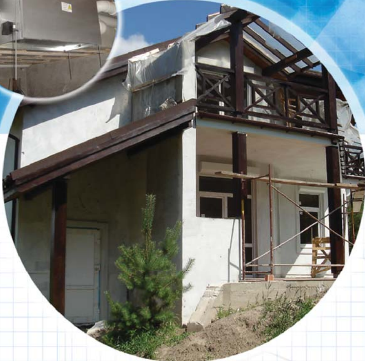
RESIDENTIAL BUILDING Kyiv Region
