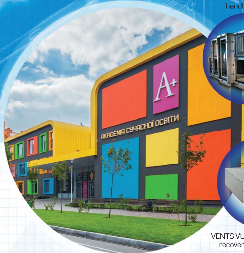
MODERN EDUCATION ACADEMY A+ CULTURAL AND EDUCATIONAL FACILITY 4 v Reheneratorna St., Kyiv
