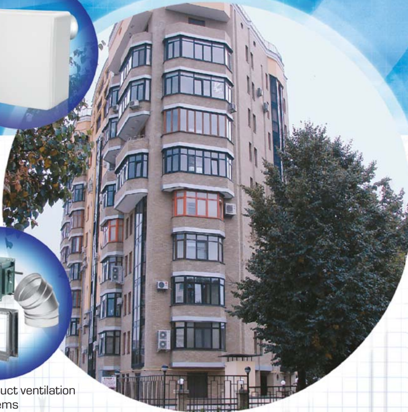
RESIDENTIAL BUILDING 18 Otakara Yarosha St., Kharkiv
