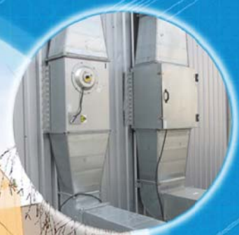
VENTS VKM and VKPF series centrifugal fans
