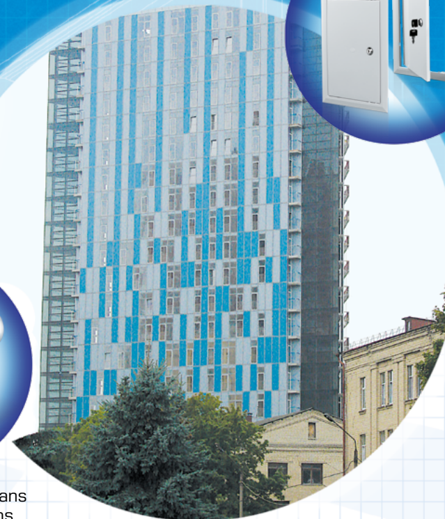
RESIDENTIAL BUILDING 18 a Otakara Yarosha St., Kharkiv
