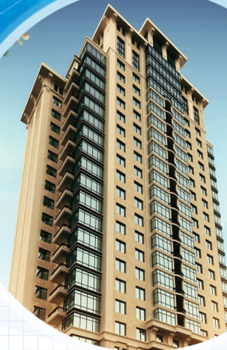
CHELSEA TOWER RESIDENTIAL COMPLEX
