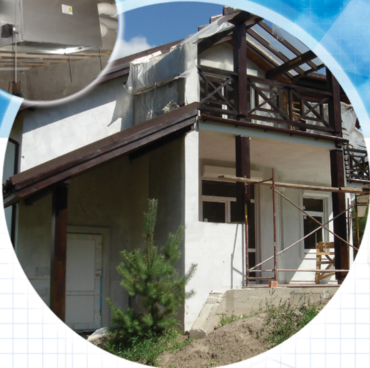
RESIDENTIAL BUILDING Kyiv Region
