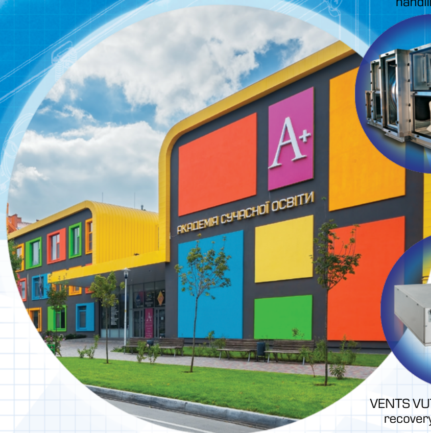
MODERN EDUCATION ACADEMY A+ CULTURAL AND EDUCATIONAL FACILITY 4 v Reheneratorna St., Kyiv
