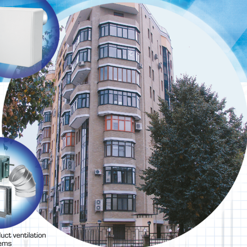
RESIDENTIAL BUILDING 18 Otakara Yarosha St., Kharkiv
