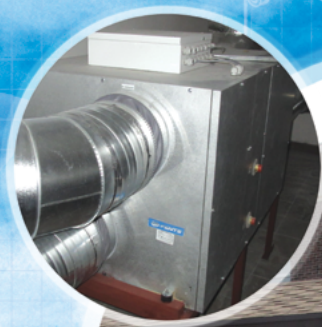
VENTS VUT R VH EC series air handling units
