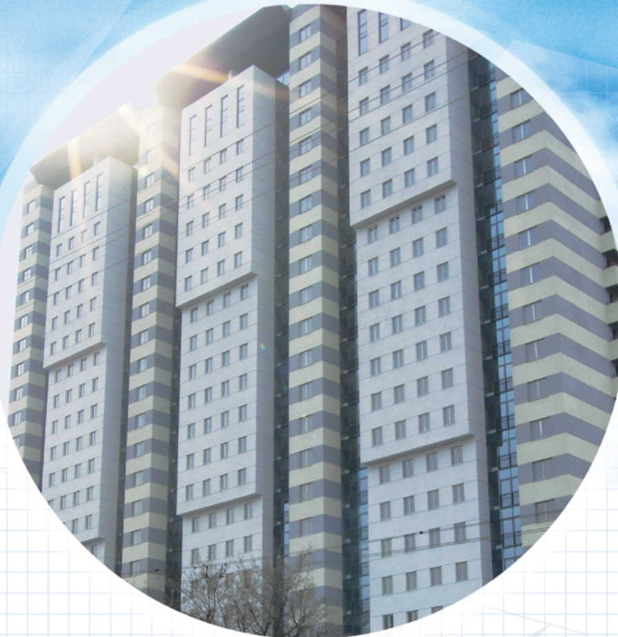
RESIDENTIAL BUILDING 18 a M. Loyana St., Dnipro
