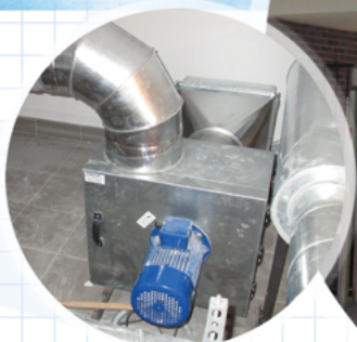
Air handling system based on VENTS KSK series fan
