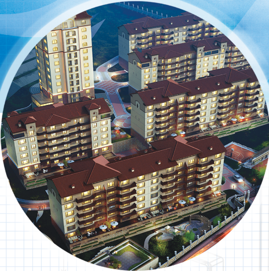
JARDEN RESIDENTIAL COMPLEX Ulaanbaatar, Mongolia
