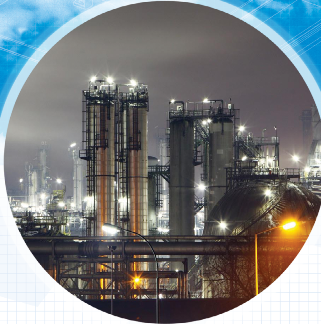
DYO PAINT FACTORY Izmir, Turkey
