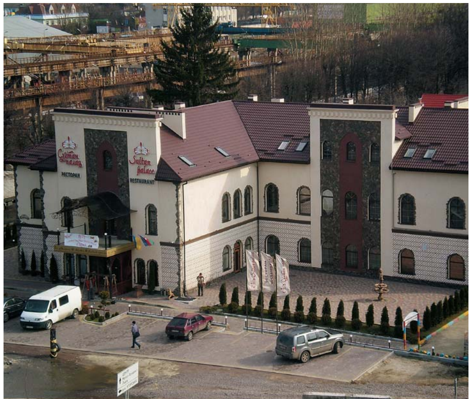
Sultan Palace restaurant, Lviv, Ukraine Air handling unit, X-Vent system
